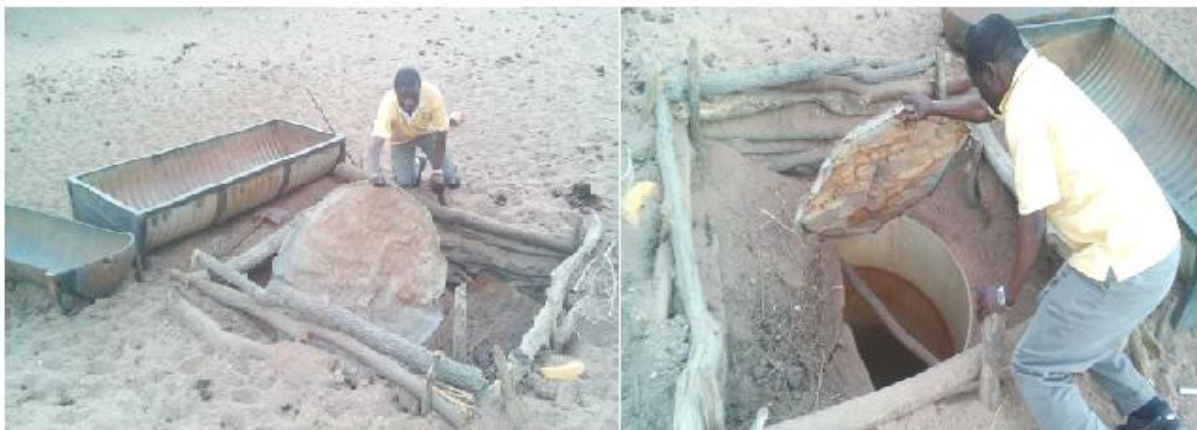
Figure 3.2: Hand-dug well in the Sedibe non-perennial river, Botswana.
