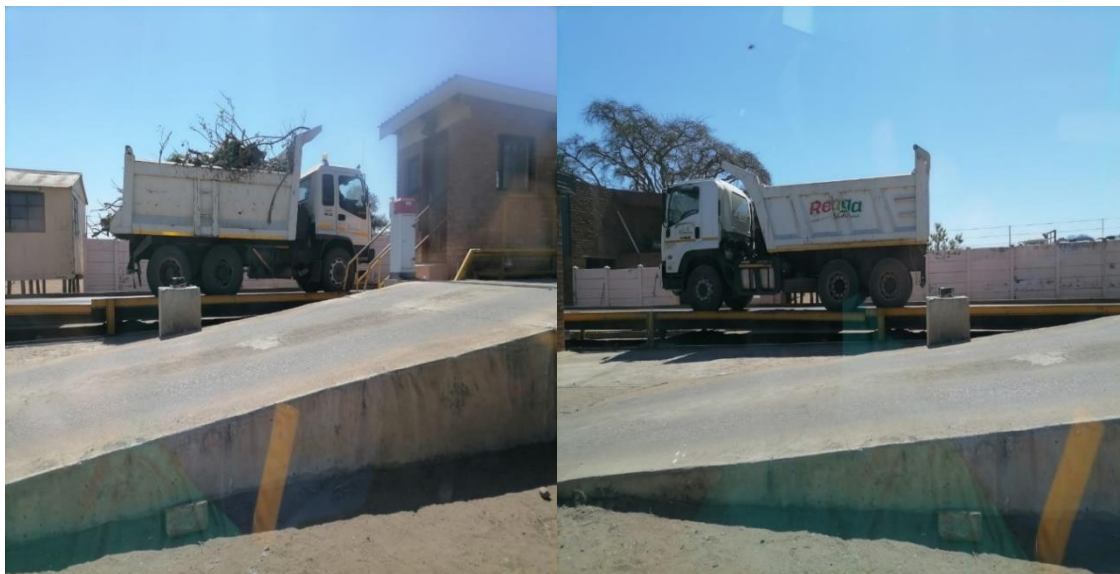
Figure 4-12: Weigh bridge at the Weltevreden landfill site
