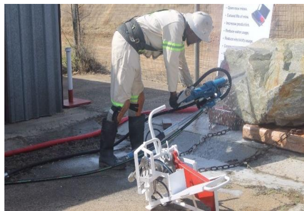
Figure 3-7: Hydropower drill demo
