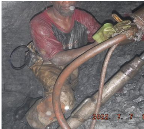
Figure 3-47: Compressed air RDO full of grease 26
