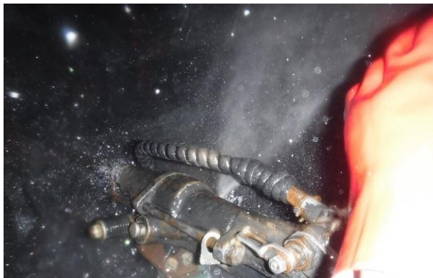
Figure 3-45: Dump hose to be connected to the drill's exhaust port 24
