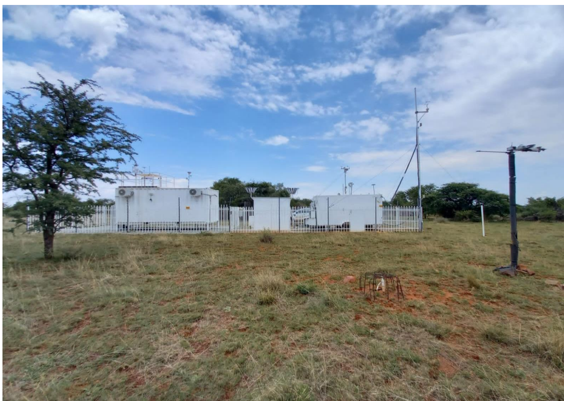
Figure 3-2: Welgegund measurement station during the summer season.
