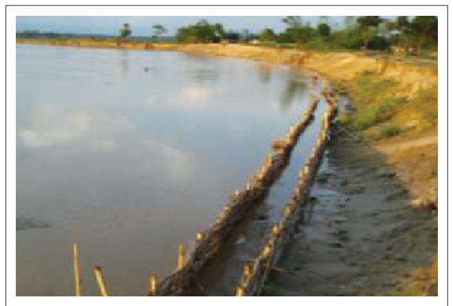
FIGURE 4: Bamboo crib wall constructed to prevent bank erosion in Nepal.
