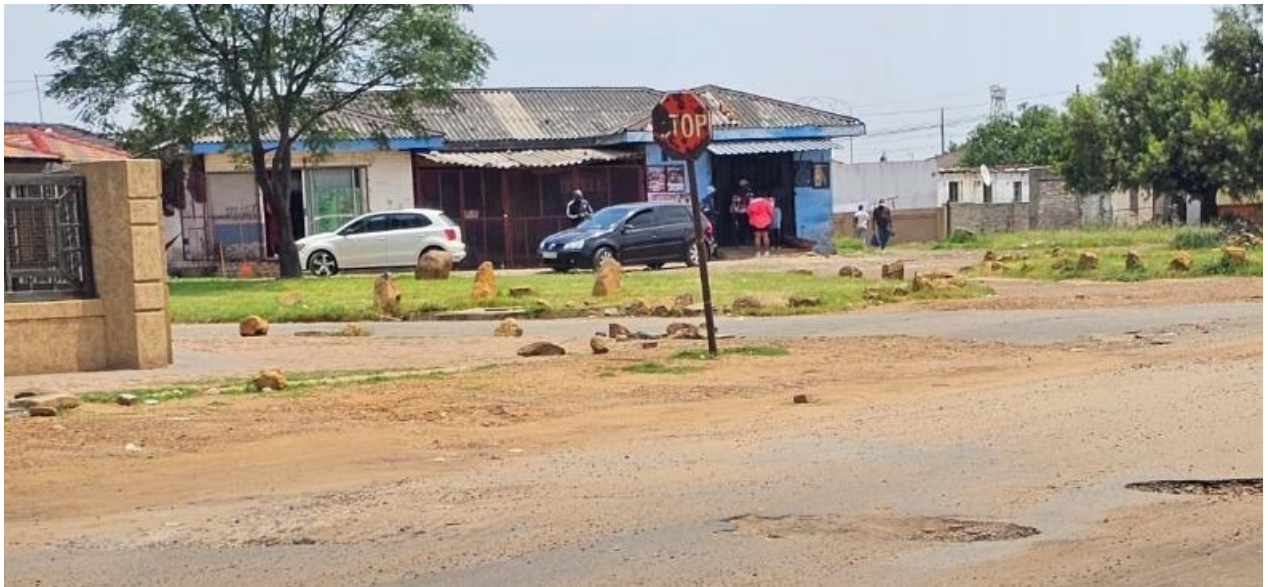
Figure 4.7: An old bathroom refurbished into a shop, Sharpeville 101
