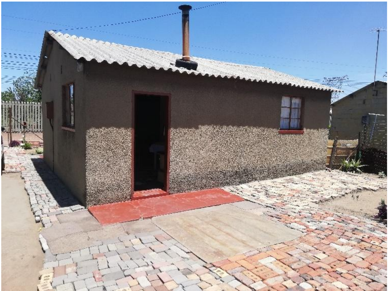
Figure 4.5: An old asbestos roof house in Vuka, Sharpeville 58
