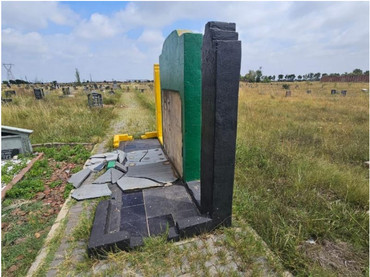
Figure 6.6: A Vandalised stone of remembrance in Phelindaba Cemetery, Sharpeville 180
