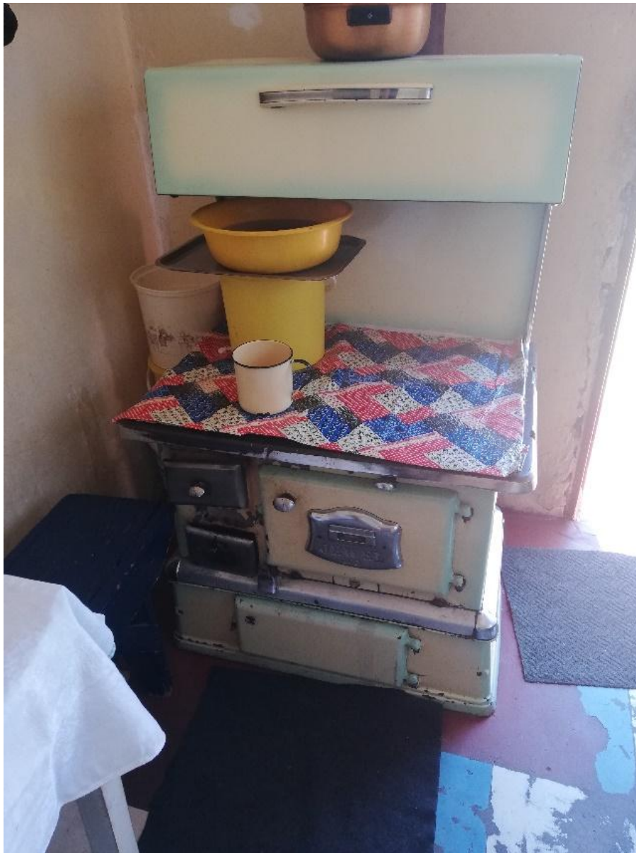
Figure 4.4: A No. 6 Dover coal stove installed in a Sharpeville house 56
