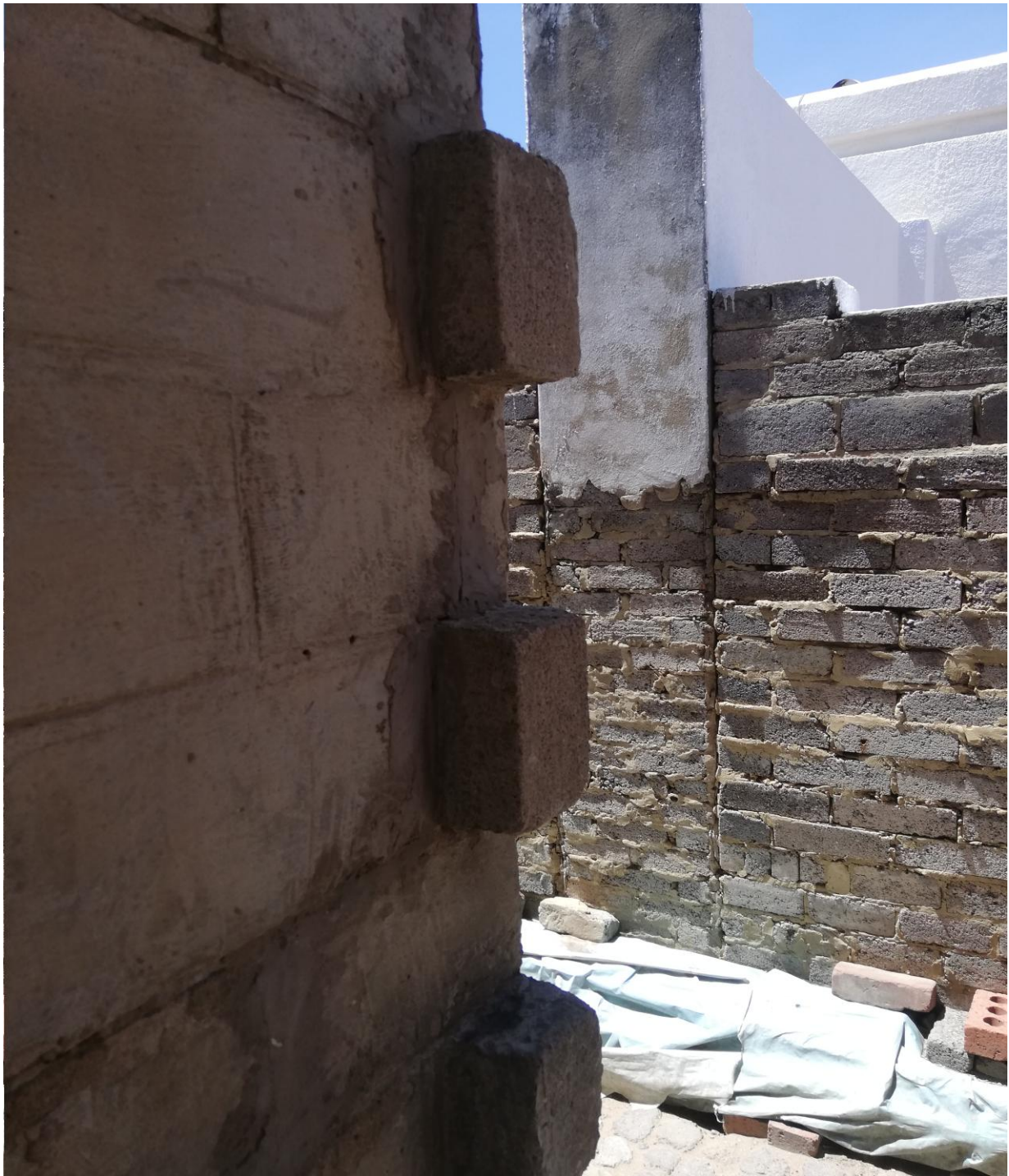
Figure 5.5: An add-on to a house constructed by the council showing where construction ended 92
