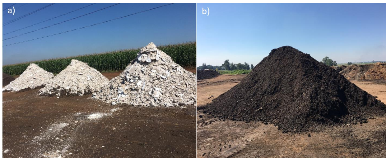
Figure 2-4: In-field mixing of organic matter with gypsum wallboard (a). The original organic material used in the mixture (b).
