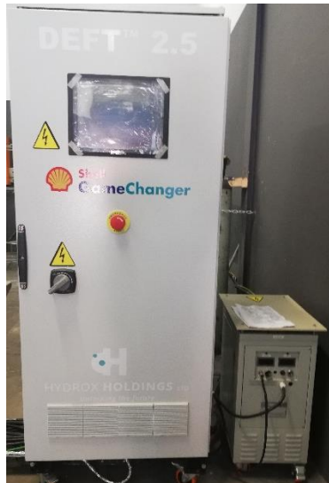
Figure 5-6: Images of the a) Electrolyser stack and BOP of DEFT™ 2.5 unit, b) scrubber units for product gases, c) gravitational separator, d) back of DEFT™ 2.5 plant - sampling panels, condensate drain, magnetic strainer and heat exchanger, e) Scada screen, f) internal of electrical panel, g) external of control panel and rectifier, and h) electrolyser stack.
