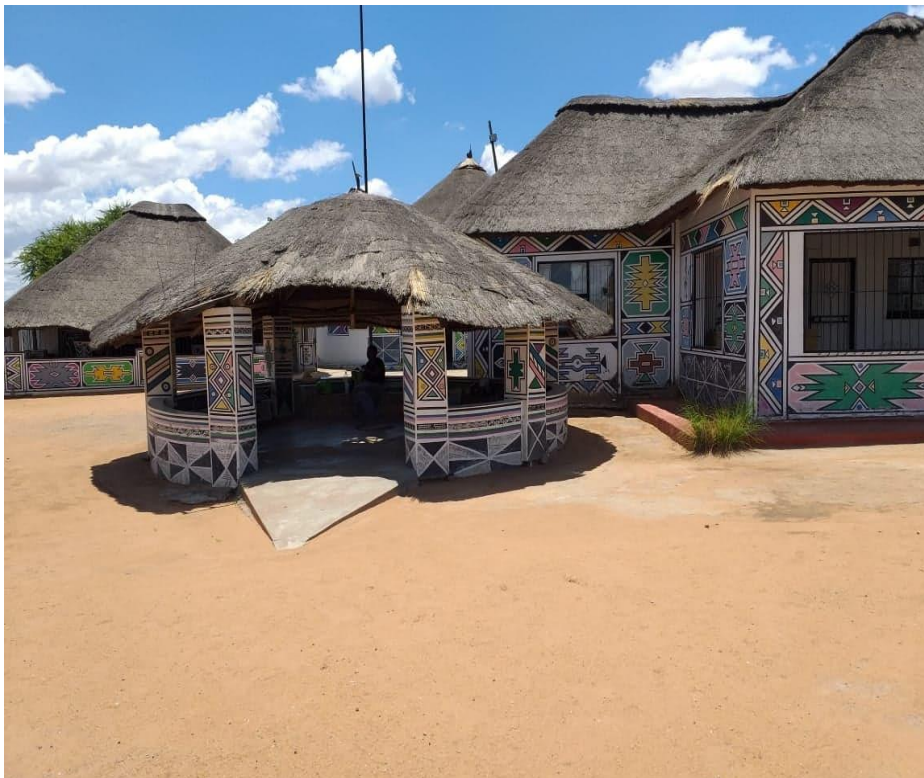
Figure 5.3: A circular structure built at ebaleni setting where women practice and transmit ethnomathematical knowledge.
