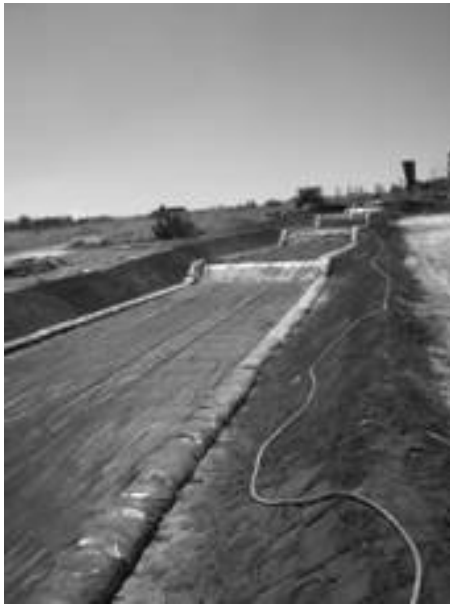
Figure 2-14: Cascades on the mine
