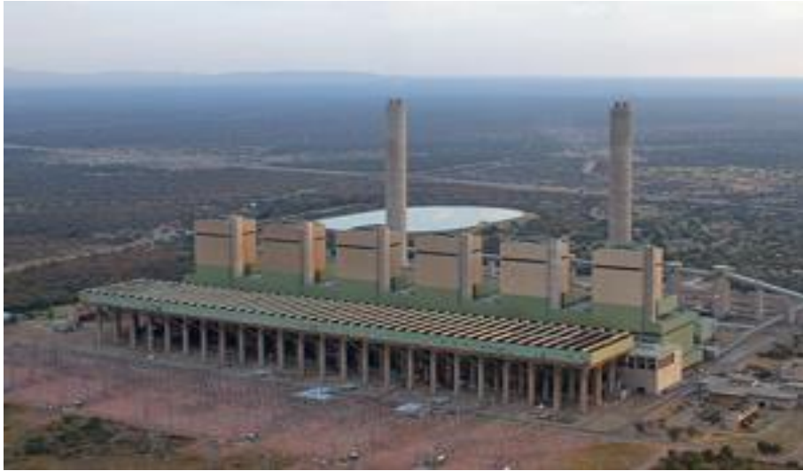
Figure 2-1: Matimba power station.
