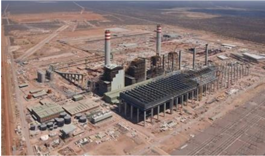
Figure 2-2: Medupi power station.
