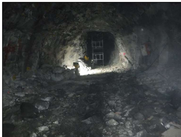
Figure 3-23: Condenser chamber with shotcrete
