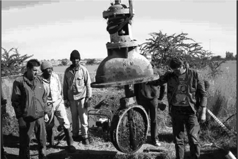
Figure 7: Removal of valve body
