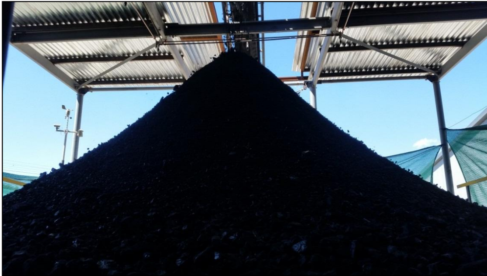
Figure 3.5.1: Experimental stockpile platform
