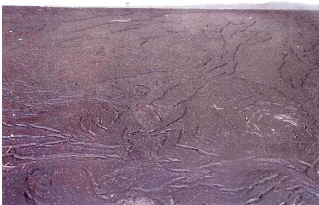
Figure 12: Treated ASP sludge in drying beds
