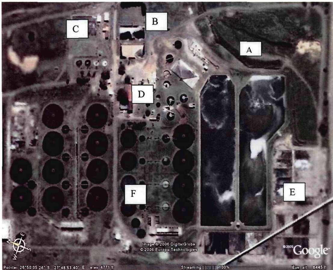
Figure 3: Physical location of process equipment A, B, C, D, E and F as illustrated in Figure 2 (GOOGLE EARTH, 2006)
