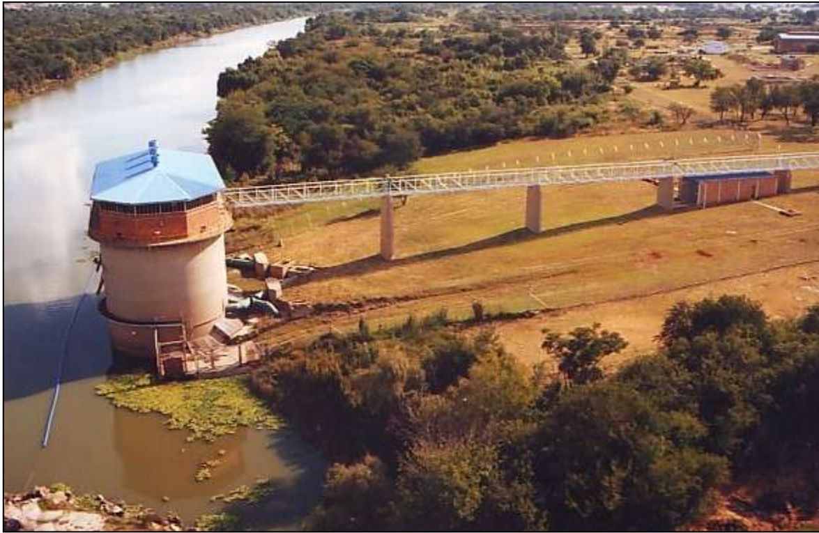
Photo 3: Intake 2 of water from the Vaal River at Midvaal Water Company, WSP for the City of Matlosana
