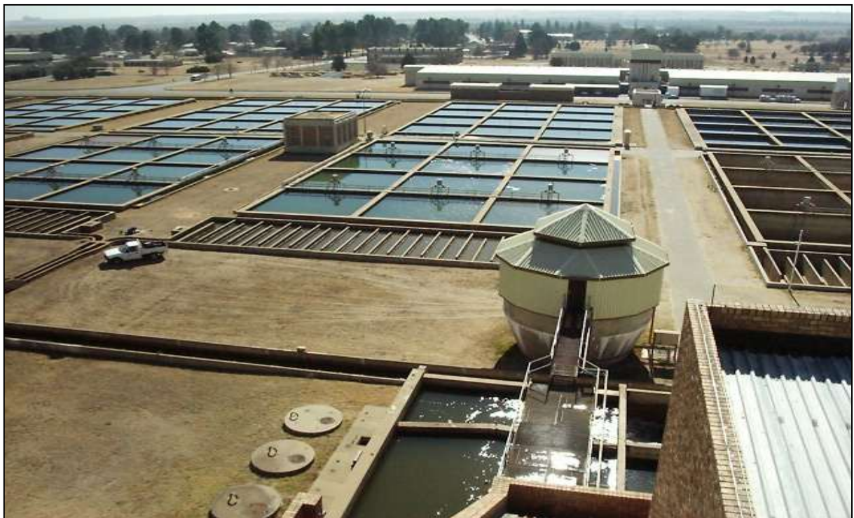
Photo 1: Water treatment works at Sedibeng Water Company, WSP for Maquassi Hills Local Municipality
