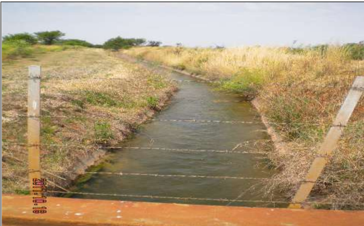
Photo 5: Open-on top cement canals transporting water destined for consumption by Potchefstroom residents
