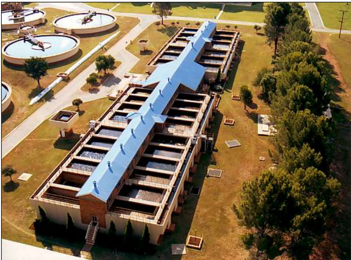
Photo 2: Water treatment works at Midvaal Water Company, WSP for the City of Matlosana
