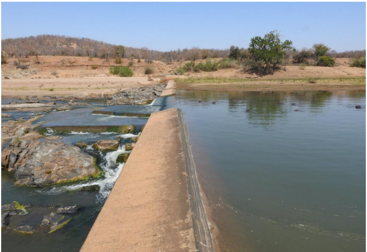
Figure 3.29: Mamba weir located upstream of Mamba study site along the lower Olifants River within the Kruger National Park.
