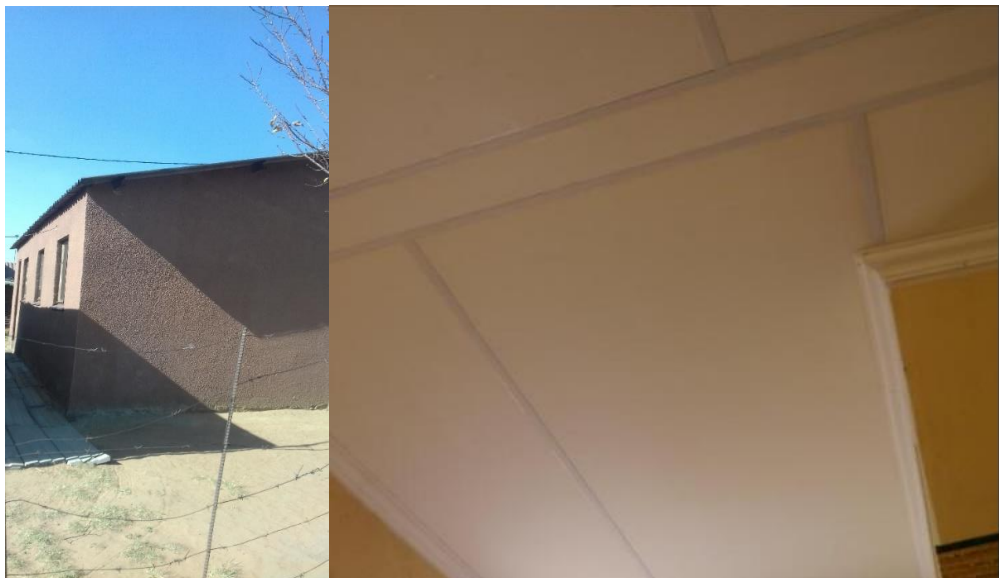
Fully insulated dwellings with northern outside elevation painted black and the inside
