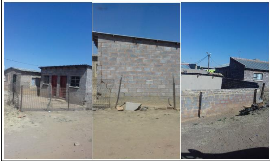
Figure 3.3: Image showing examples of sampled RDP residential dwellings in KwaZamokuhle (Source: Matandirotya 2017)
