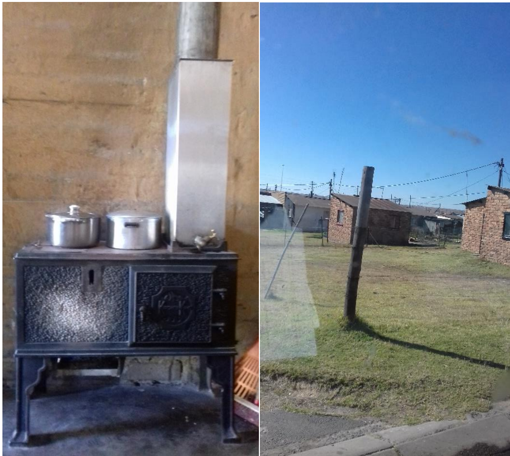
Typical coal stove used in low-income dwellings
