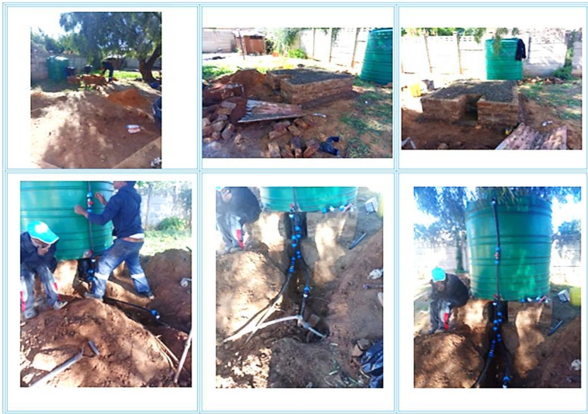
Figure 6.3 JoJo tank installation
