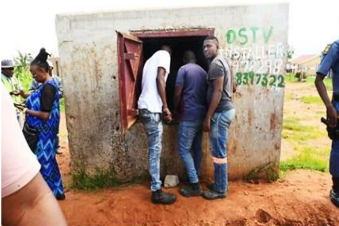
Figure 3.2 Polokwane Local Municipality illegal water connection
