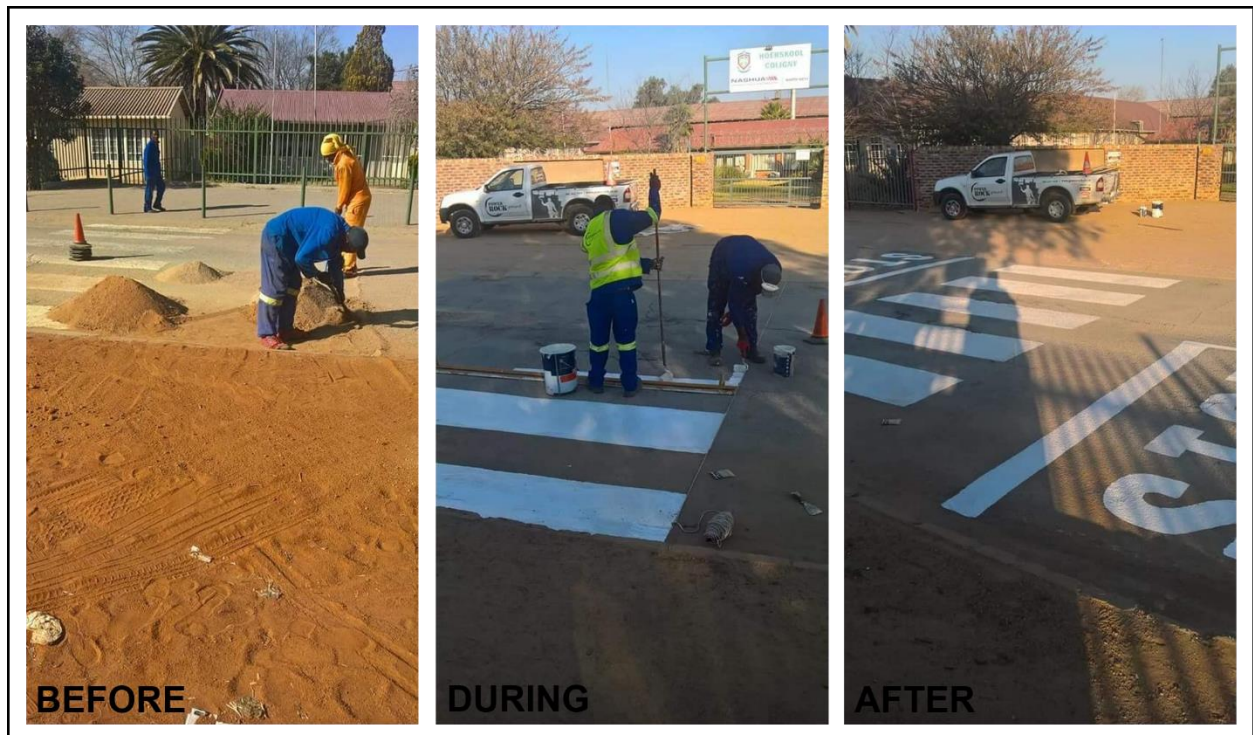
Figure 4-8: Coligny Forward project before and after road signage painting
