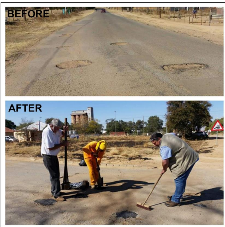
Figure 4-7: Coligny Forward project before and after road and pothole repairs
