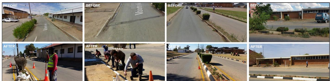
Figure 4-5: Coligny Forward project before and after curb painting
