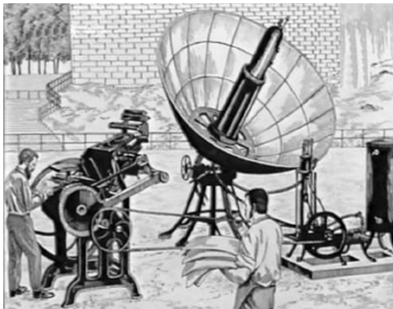
Figure 2-32: Historical use of solar power in printing press (Gevorkian)
