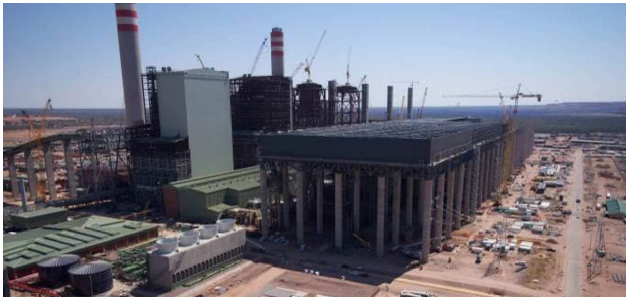
Figure 2-58: Medupi power station construction site (Eskom, 2014b).
