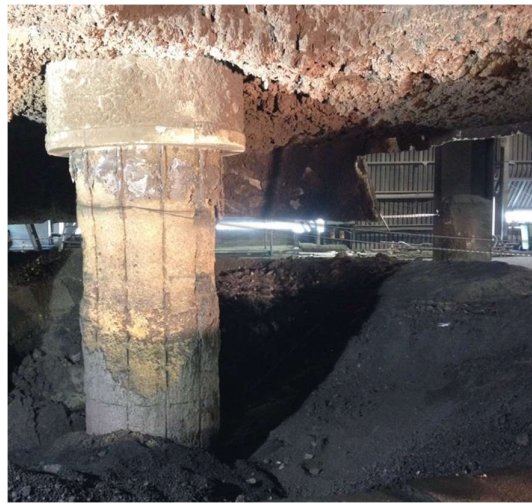
Figure 3.3 Photo indicating how Electrode 2 from Furnace 3 was cut off, approximately 0.5 m below the contact shoes with a diamond-coated wire saw.
