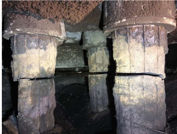
Figure 3.4 Upright, post-cut electrodes from Furnace 1 that is being held up by the raw material mixture.
