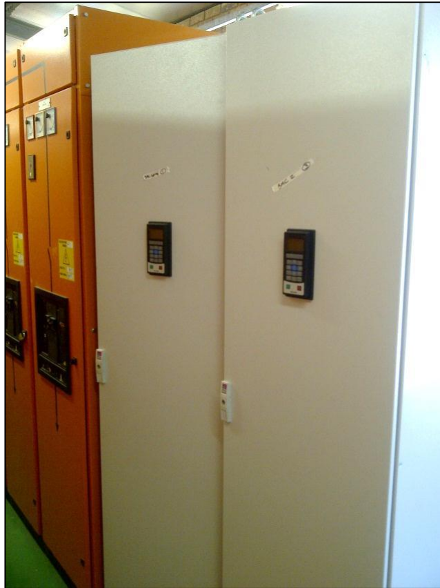
Figure 81: VSDs installed on the BAC spray pumps.
