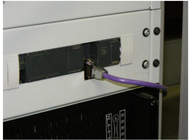
Figure A.6 – PLC PROFIBUS interface
