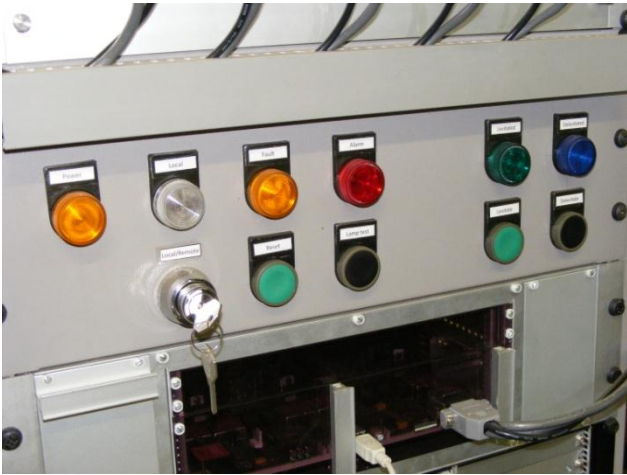
Figure A.5 – PLC interface
