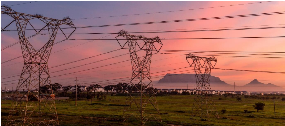
Figure 71: High-voltage power lines 76
