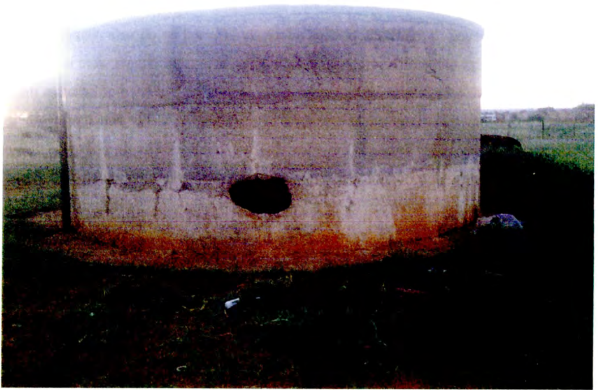
This dam used to store and supply the community with water generated through the windmill
