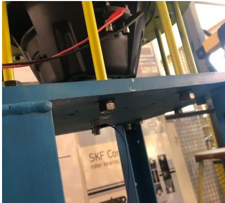
Figure 5-2 PCB sensor mounted
