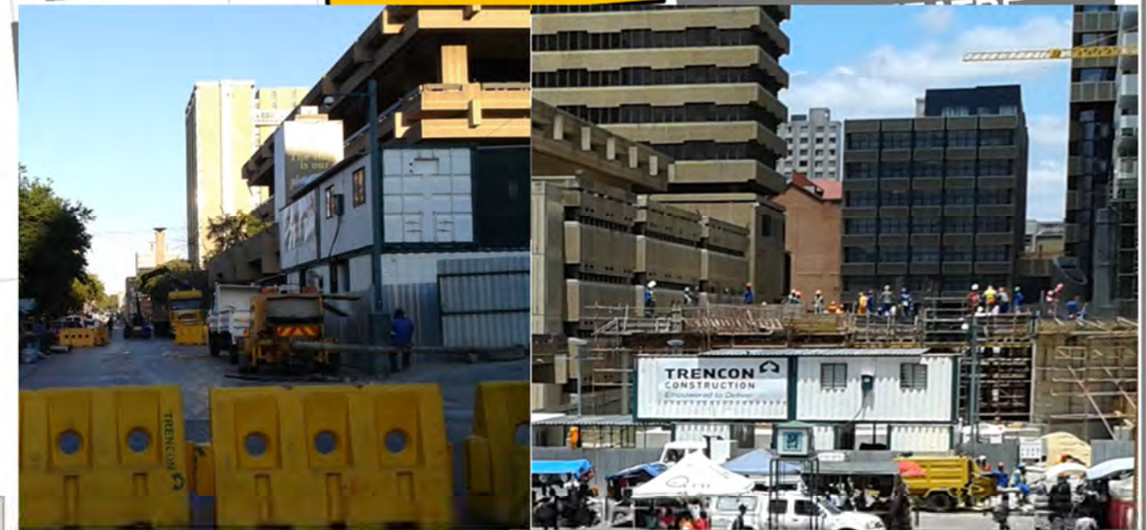
(E) Lilian Ngoyi Square currently under construction (Source: Photograph taken by researcher)
