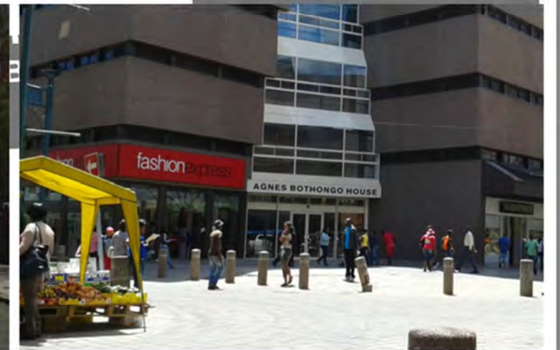
(F) Buildings on erf boundary that line the street with an active frontage (Source: Photograph taken by researcher)
