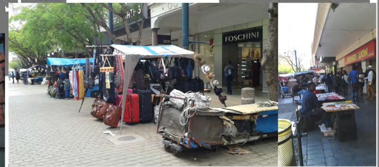
(D) Informal trader stalls act as a barrier in front of building facades, creating a narrow sidewalk (Source: photographs taken by researcher)
