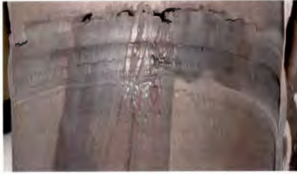
Fig. 6(b): Intergranular corrosion on the heat-affected zone of a circumferential weld.
