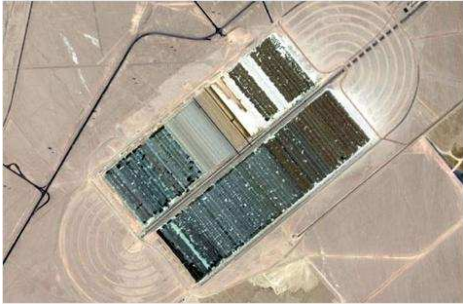
Figure 2.2: The OOHLP layout or also referred to as the race track (FLSmith website – conveyor section (Nov 2011)).
