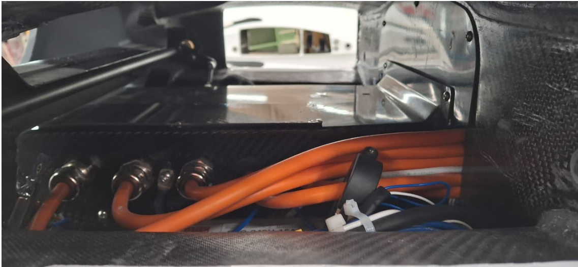
Figure 3.8: Complete motor-controller assembly inside the fuselage (side view, airflow from left to right)
