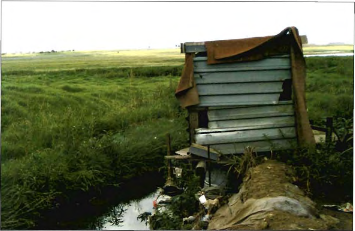
Figure 6.6: Pit toilet made next to the stormwater channel in Harry Gwala
