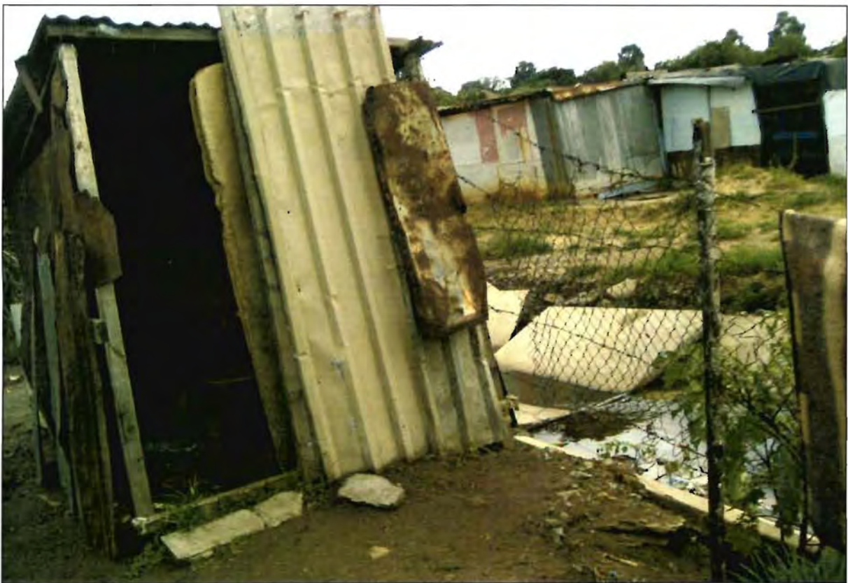
Figure 6.7: Pit toilet made next to the stormwater channel in Harry Gwala
