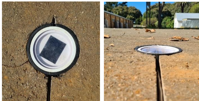
Figure 5-31: The in-road sensor installation (-26.6943, 27.0900)
