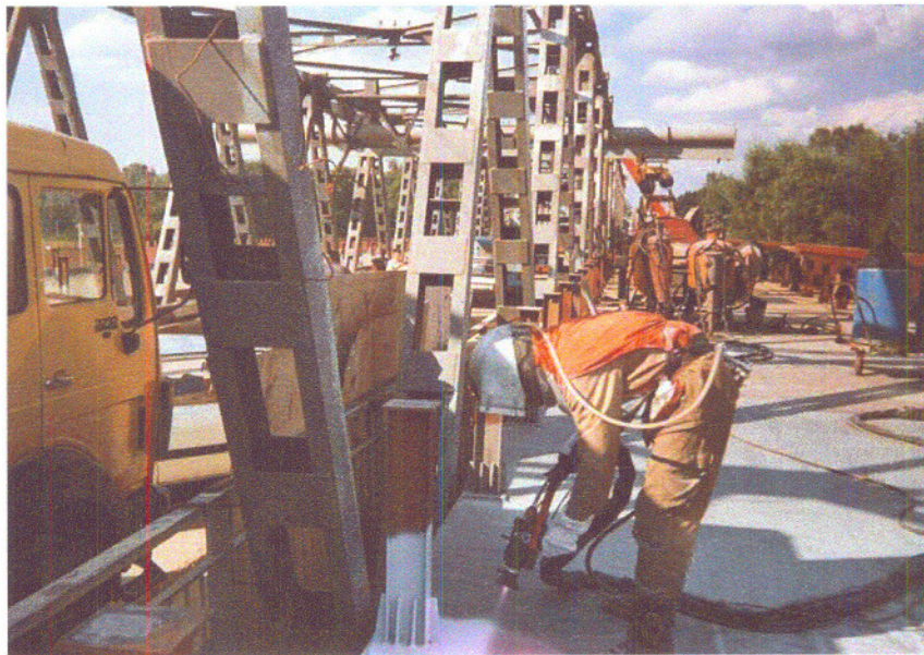
Figure E.12 Metal spraying with the HVAF gun
