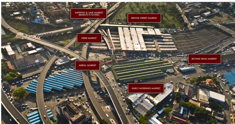
Figure 5-27: Warwick junction renewal pilot project
