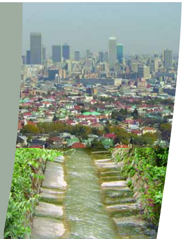
Johannesburg Canalised stream running through Johannesburg
