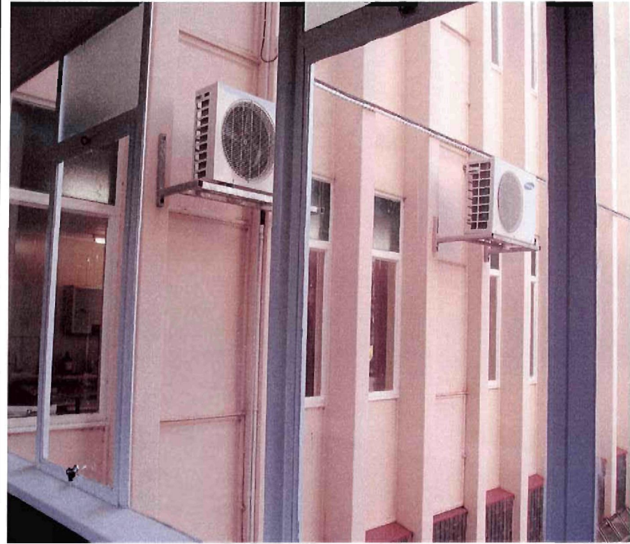
Figure A.18 View of facility relative to adjacent corridor. Angled outer view of laboratory/site opposite the door entrance.
