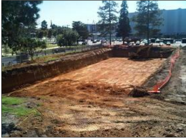
Figure 33: Kardinia Park, construction of underground storage tanks Source: Clearwater (2012)
