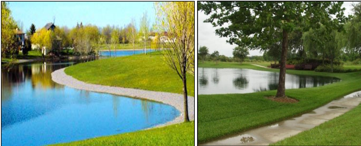
Figure 21: Retention Ponds. Source: Lakeside Design service (2012).
