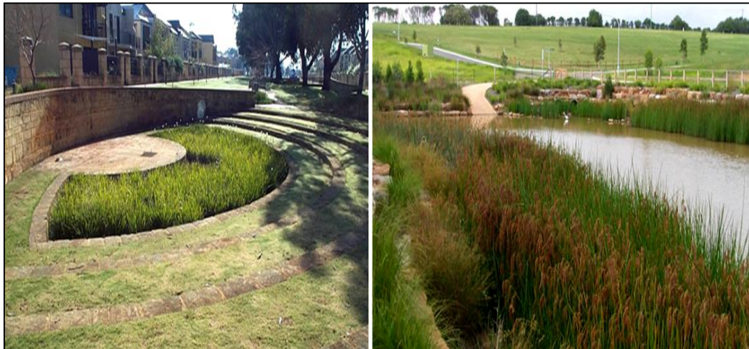
Figure 18: Constructed Wetlands. Source: Water Sensitive Urban Design (2012).
