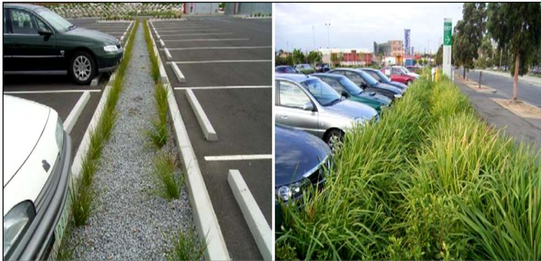
Figure 19: Infiltration trenches surrounding car parks Source: Water Sensitive Urban Design (2012)
