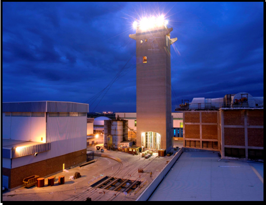
Photo: By HVAC International personnel
