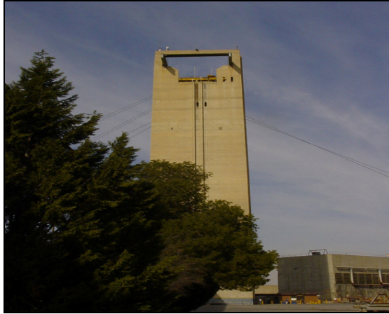
Figure 14: Photo of Masimong 4# gold mine
