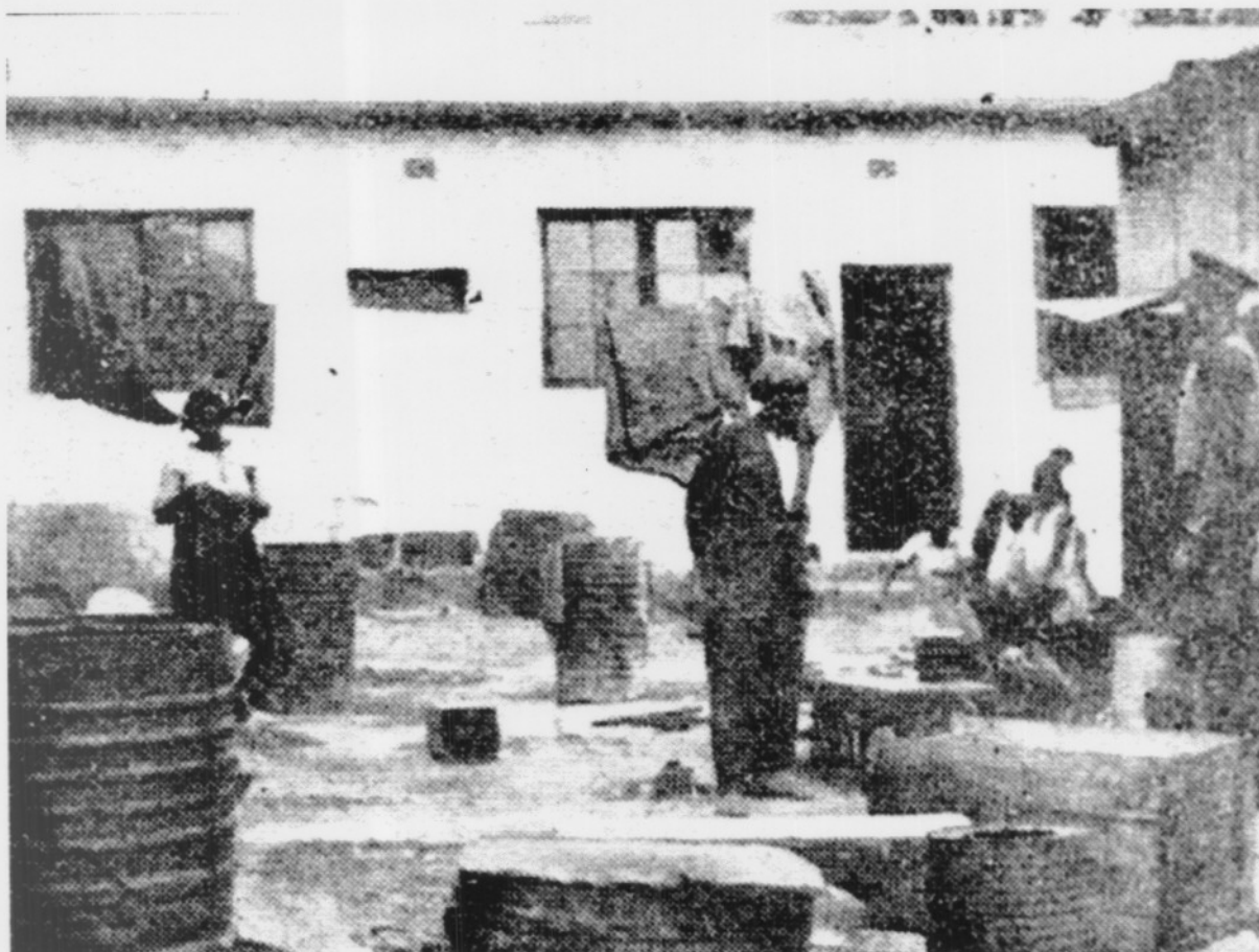
A Johannesburg yard. The drums were used for storing water or for cooking food. Overcrowding, poverty, and the lack of services – clean water, sewerage and rubbish collection – were major causes of disease.
