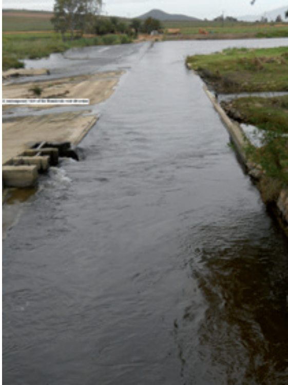
Image 2: A contemporary view of the Bonnievale weir-diversion
