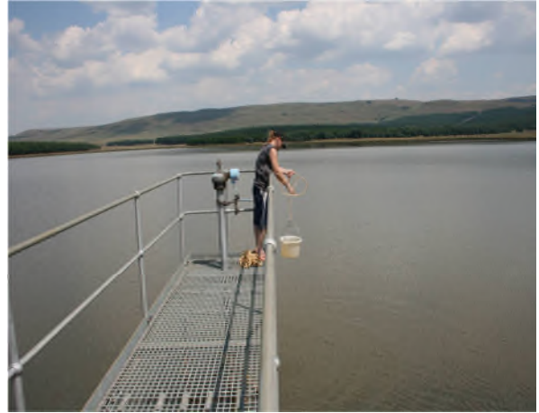
PLATE 4.2: Monitoring site GHB-Q01 at the pipe outlet at Geelhoutboom Dam.
