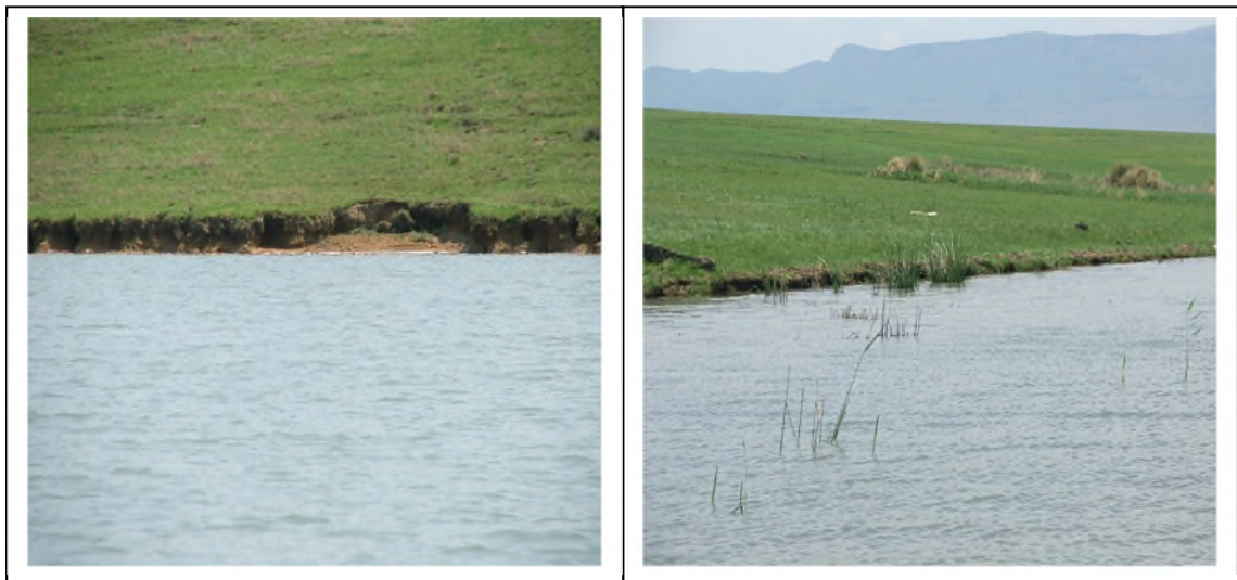
PLATE 5.10: Typical eroded and intact open bank biotopes of Heyshope Dam.
