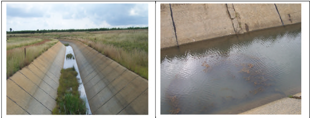
PLATE 6.1: Rushes ( Juncus sp.) (left) and Fine oxygen weed ( Lagarosiphon muscoides ) (right) causing operational problems in the Geelhoutboom Canal system.
