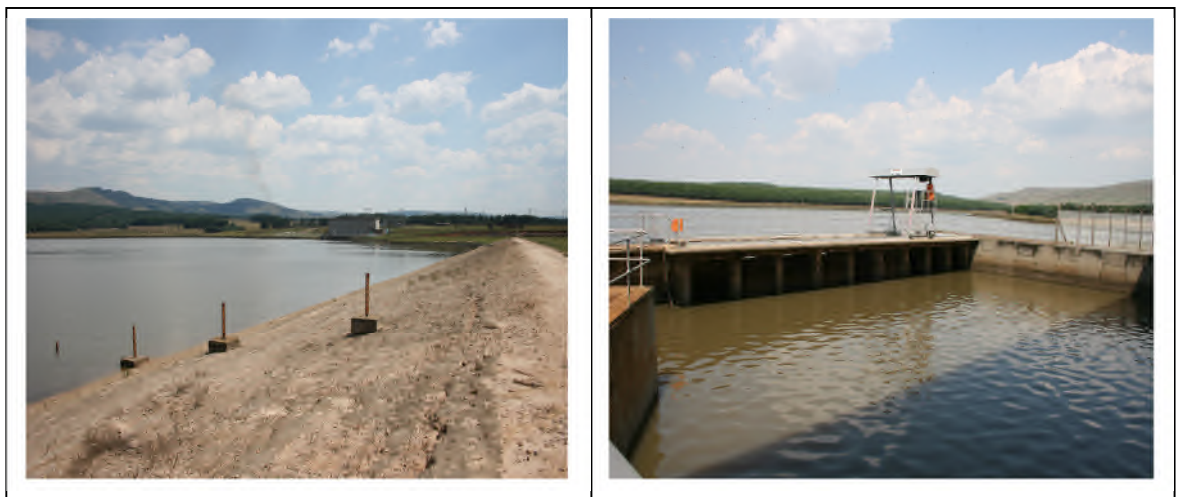
PLATE 5.22 Geelhoutboom balancing dam, dam wall with water level gauge plates on the left, and the forebay metal grids of the Geelhoutboom Pump Station on the right to prevent SAV sucked into the pumps.
