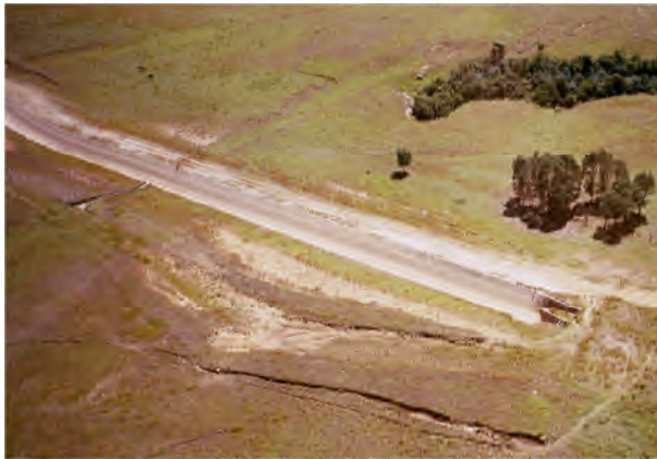
PLATE 4.3: Monitoring site GHB-IN – intake of the Geelhoutboom Canal.
