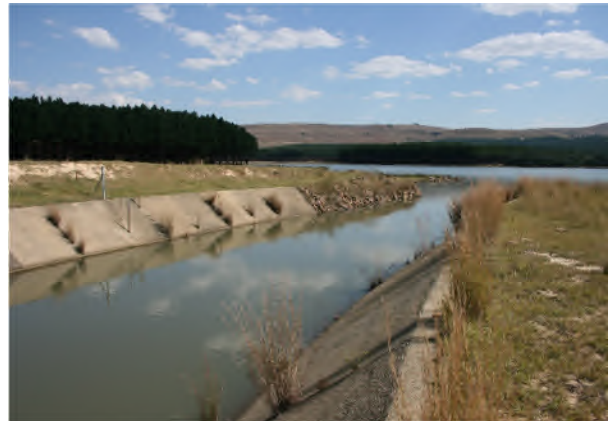
PLATE 4.4: Monitoring site GHB-OUT – outlet of the Geelhoutboom Canal into the Geelhoutboom balancing dam.
