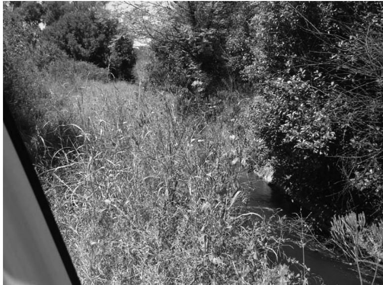
Image 3: Nature and extent of the overgrown canal and its ill-maintained servitude
