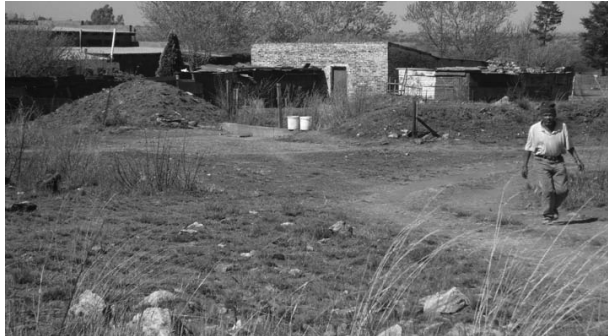
Image 4: Unlawful theft of water from the canal as well as some visible slaughtering of live stock on the cement overhang
