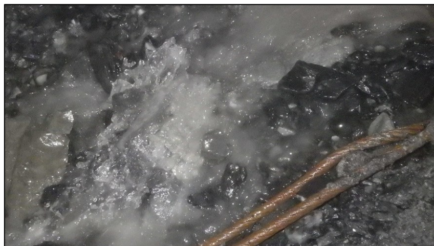
Figure 3-10: Close-up of water flowing in strike gully
