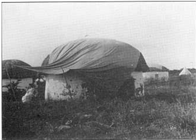
Nurse in front of Plague Camp huts, 1903. The squalor and ramshackle nature of the wattle-and-daub buildings is clearly visible.
