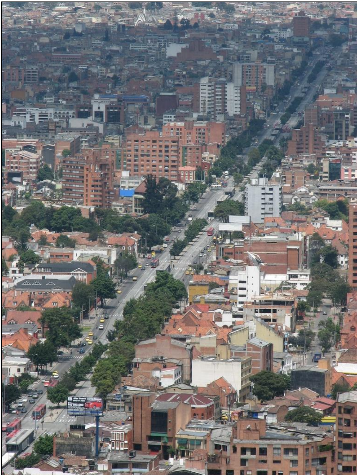
FIGURE 9 - DEDICATED BUSWAYS OF BOGOTA'S TRANSMILENIO BRT SYSTEM
