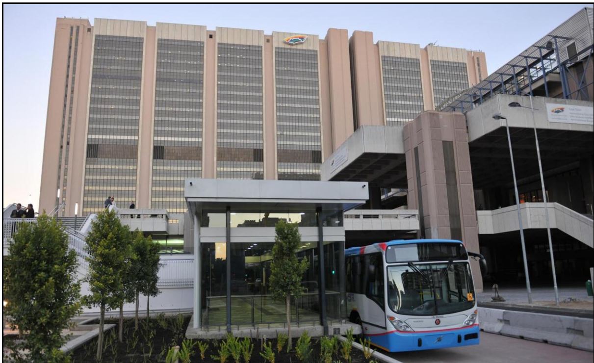
FIGURE 16 - THE COMPLETED MYCITI IRT STATION AT THE CAPE TOWN CIVIC CENTRE
