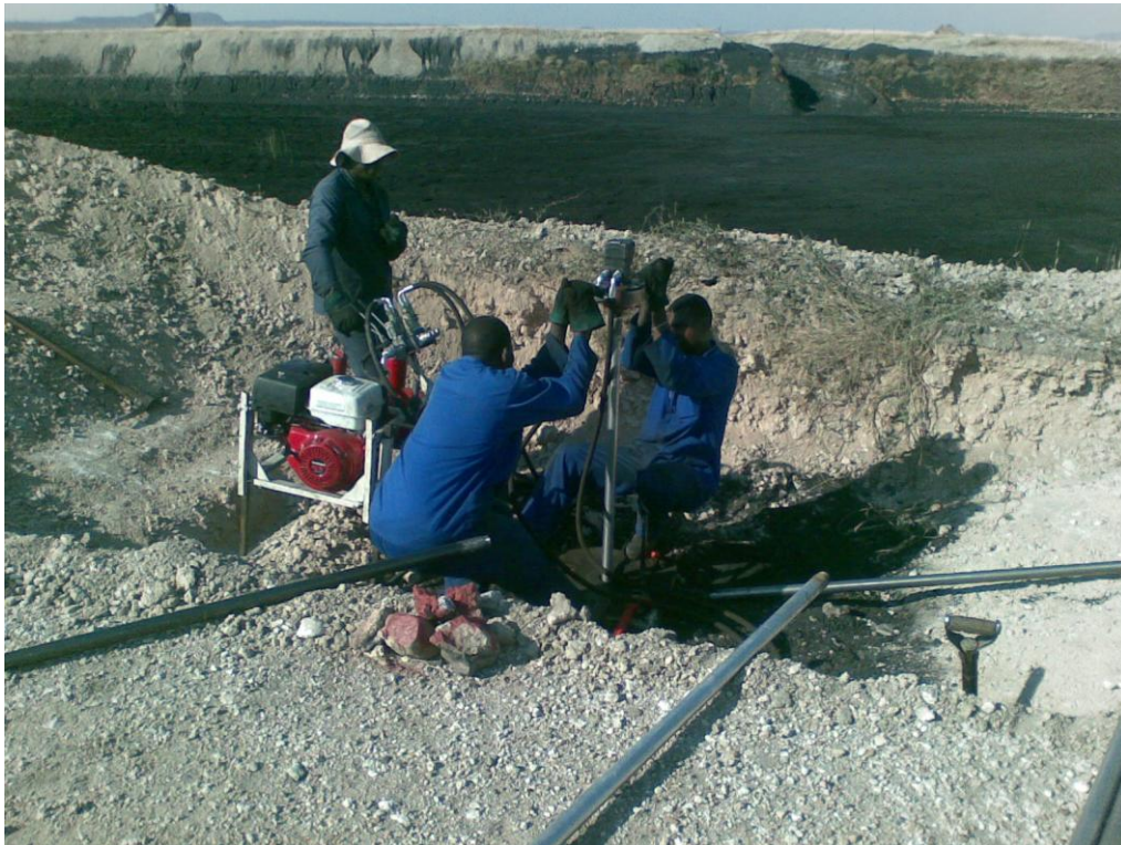
Figure 3.4: Auger drill view 1
