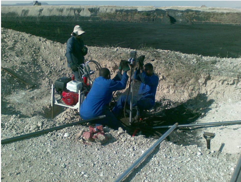
Figure 3.5: Auger drill view 2
