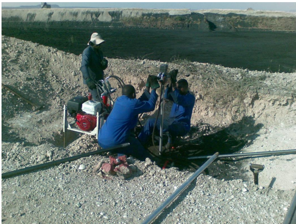
Figure 3.6: Auger drill view 3
