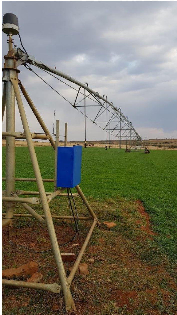
Figure 36: CPIS controller and towers.
