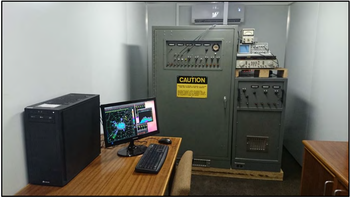
Figure 69: Radar setup inside the container
