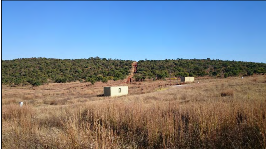
Figure 22: Path for the power cable down the hill towards the power supply on the right side
