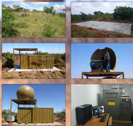
Figure 4-9: Installation process of the North West University's weather radar
