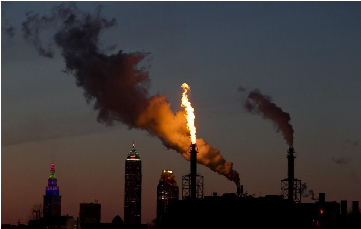
Figure 5: Steel plant active flare stack 3
